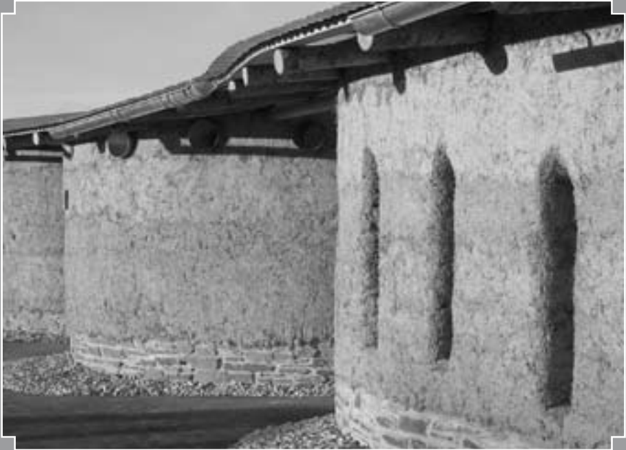
Fig. 4: Cob visitor facility, window details, Eden Project, Cornwall (J. Abey and J. Smallcombe).
